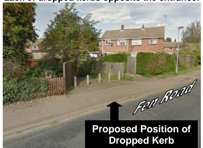
Photo 2 – Lack of dropped kerbs opposite the entrance:
